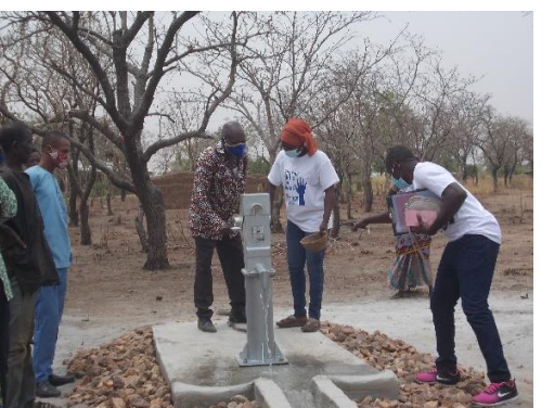
GES Director pumping the borehole
